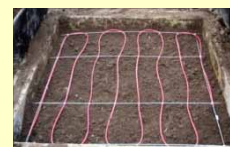
Soil warming cables at 10 cm depth
